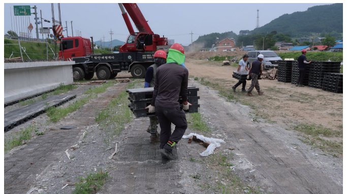
Step_7 Dismantle floor formworks
