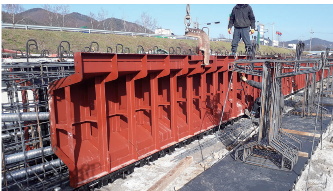
Step_4 Rebar assembly and Install steel formworks
