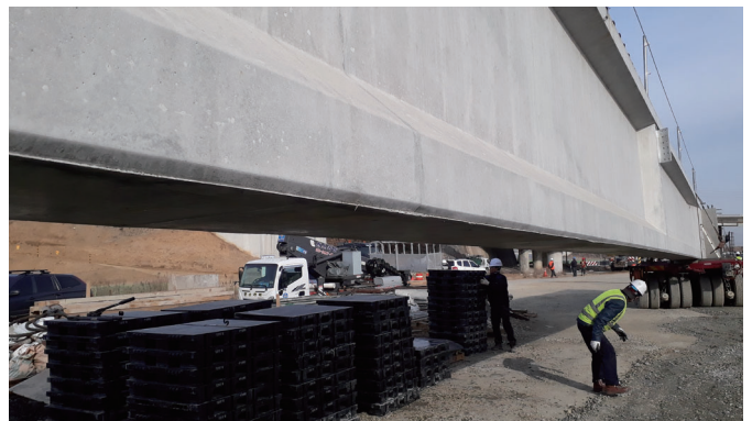
Step_6 Erection of PSC girders
