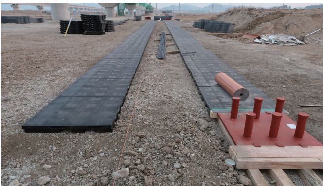
Step_3 Install floor formworks
