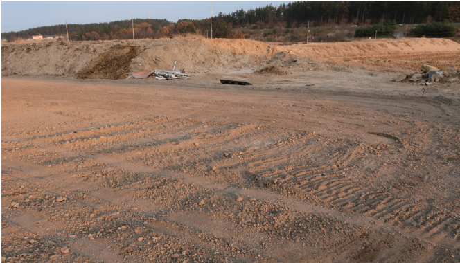
Step_1 Site preparation
