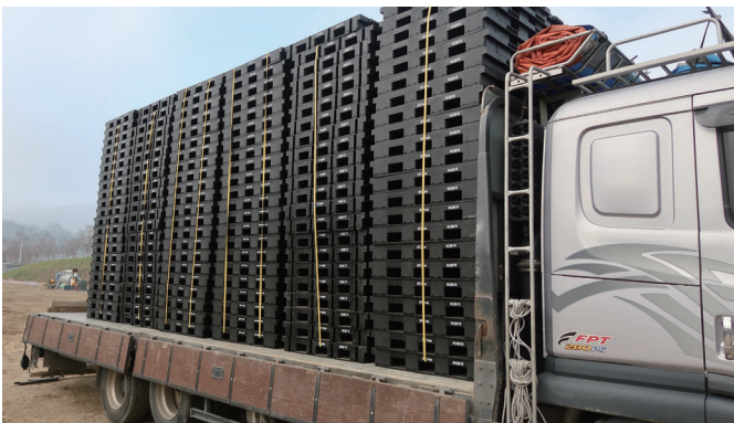
Step_2 Deliver floor formworks to site
